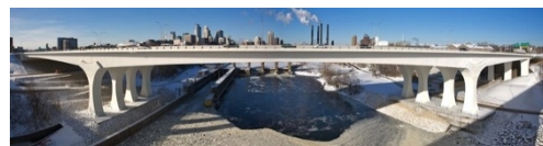
J&L provided the labor for the steel installation of the I 35W bridge project
